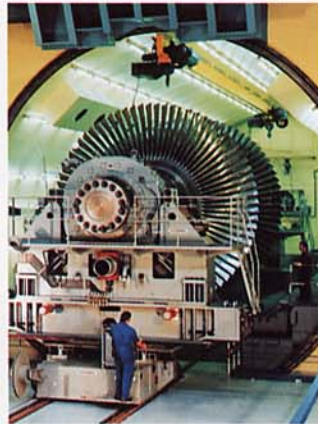
Balancing and Overspeed Test Facility DH 11 with burst protection tunnel building. An LP turbine rotor installed in the balancing pedestals is just being moved into the tunnel.
